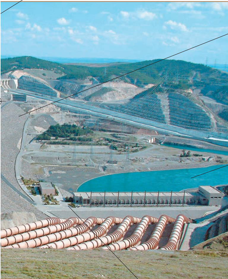
The hydroelectric power plant has 8 turbines and an installed capacity of 2400 MW
