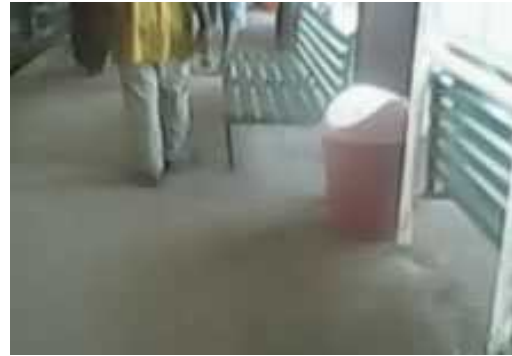
Figure4.10 Railway Station Seats
