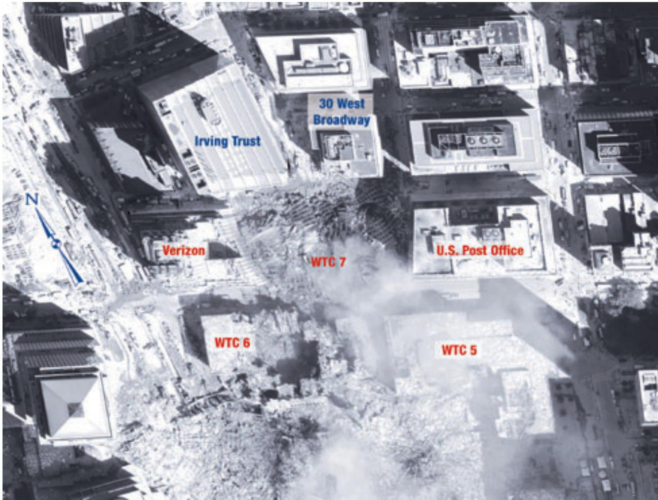
Figure 5-26 Debris generated after collapse of WTC 7.
