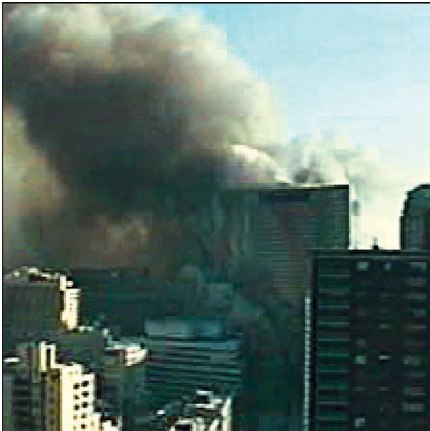
Figure 5-22 East and now west mechanical penthouses gone. (From video.)
