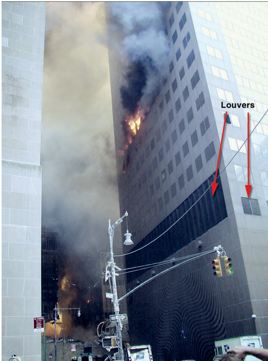
Figure 5-19 Fires on the 11th and 12th floors of the east face of WTC 7.
