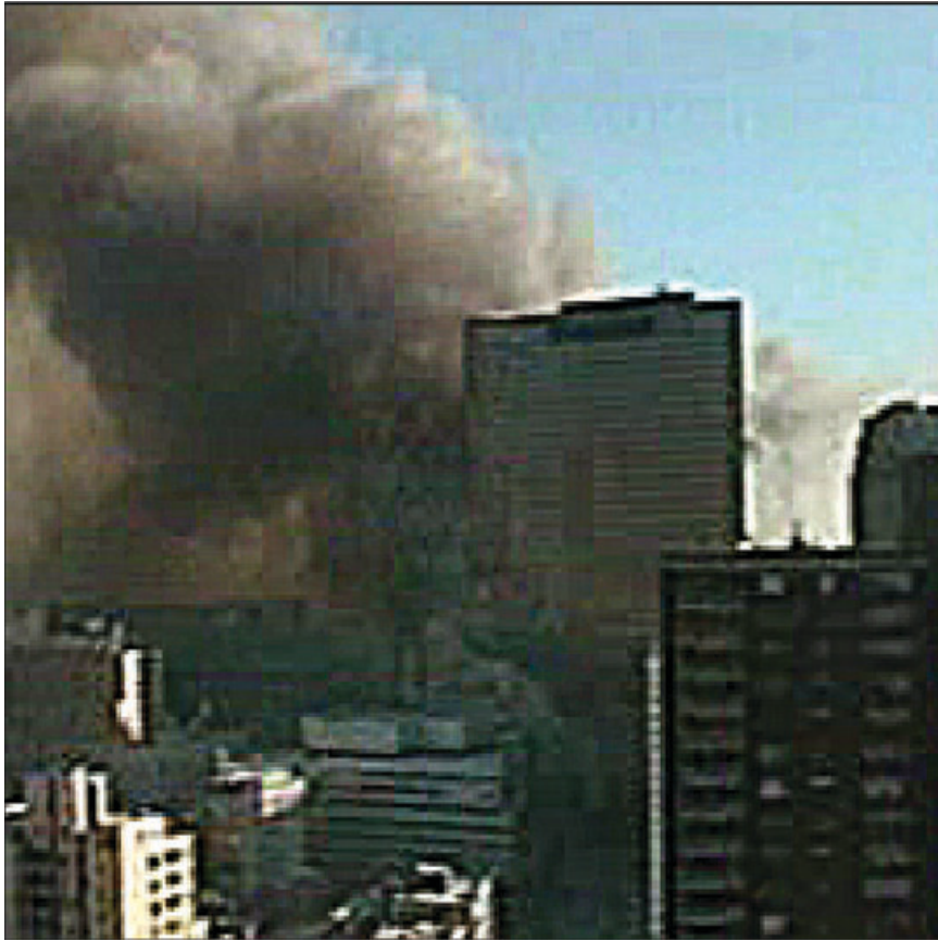
Figure 5-21 East mechanical penthouse collapsed. (From video.)
