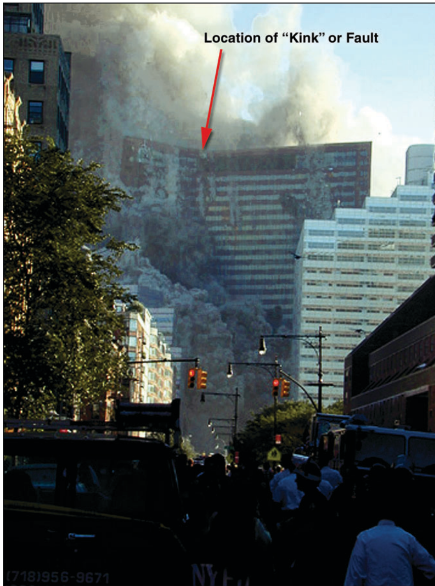
Figure 5-23 View from the north of the “kink” or fault developing in WTC 7.
