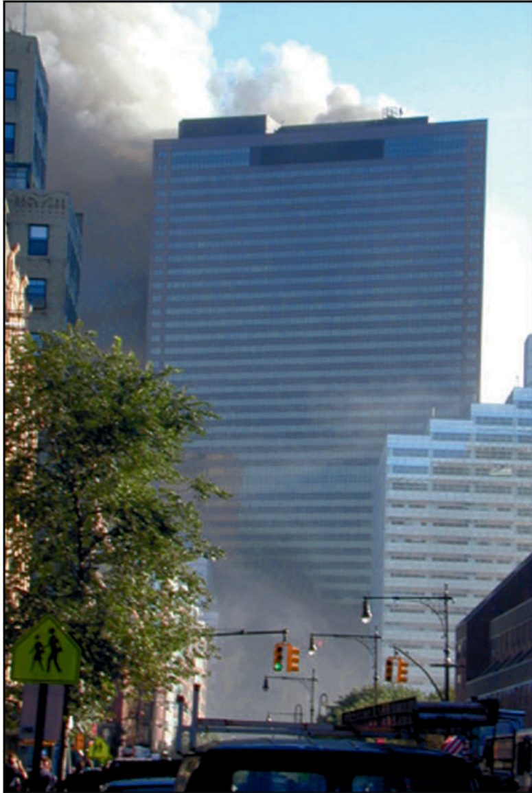
Figure 5-20 View from the north of WTC 7 with both mechanical penthouses intact.
