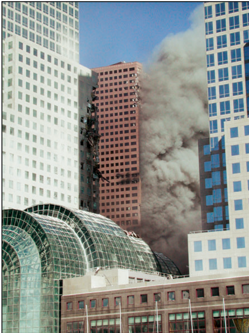
Figure 5-17 Building damage to the southwest corner and smoke plume from south face of WTC 7, looking from the World Financial Plaza. Note damage to WFC 3 in the foreground.
