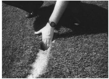
A 3-inch-wide slit drain just after installation.
