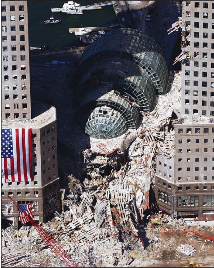
Figure 7-3 View of Winter Garden damage from West Street, with WTC 1 debris in front of WFC 2.
