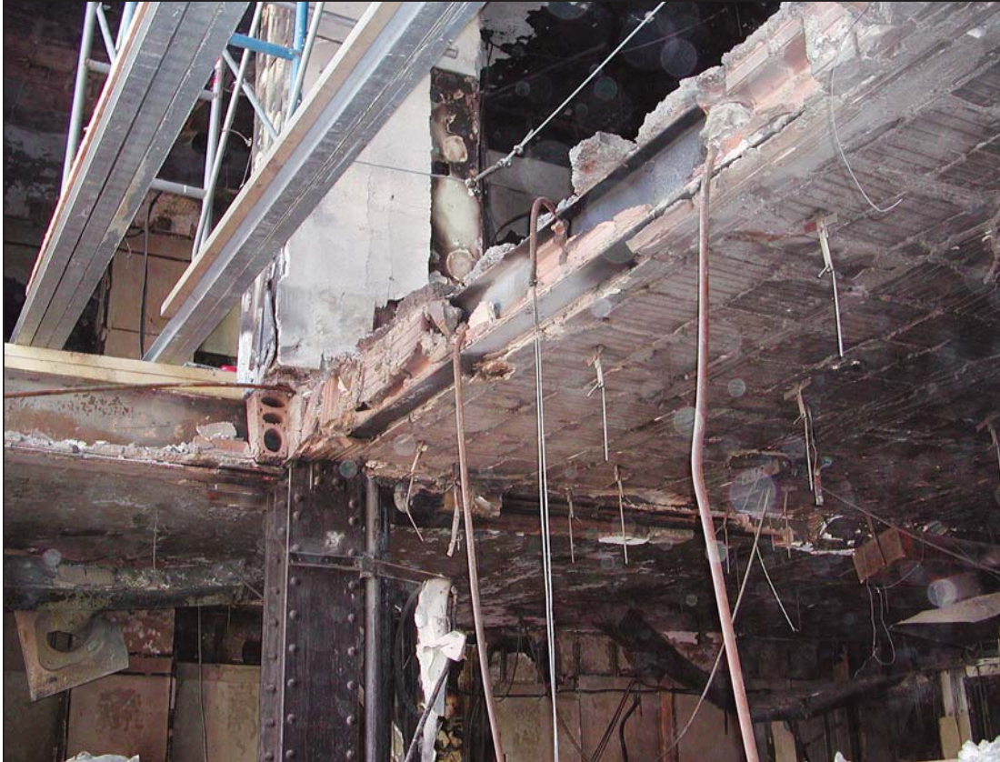
Figure 7-15 Interior of 90 West Street showing typical construction features.
