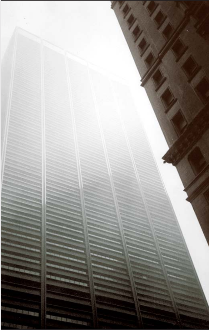
Figure 7-19 One Liberty Plaza – south elevation, upper floors.
