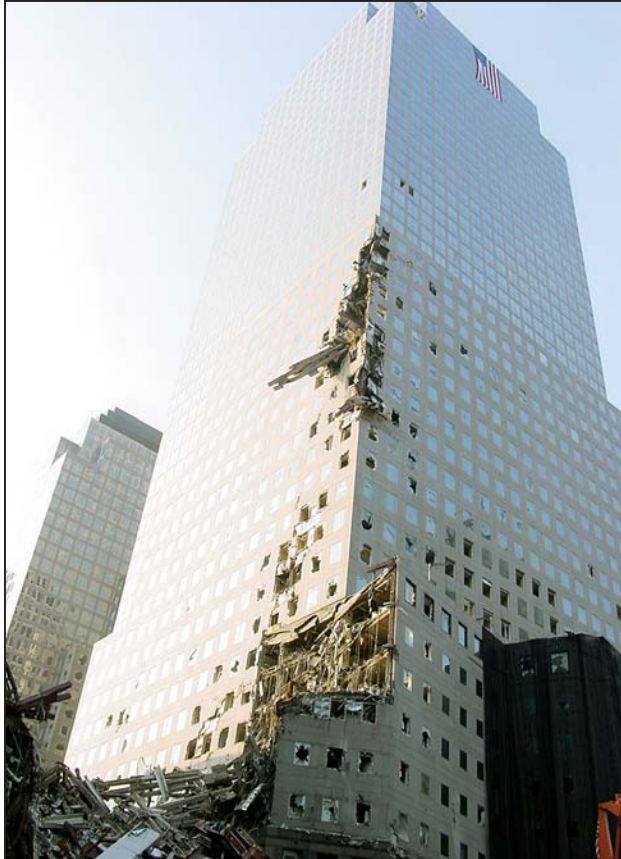
Figure 7-2 Southeast corner of WFC 3.
