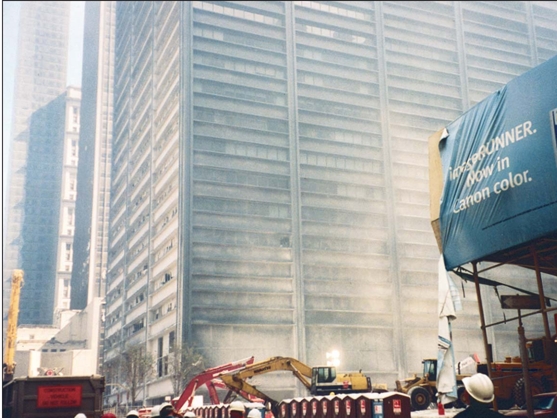
Figure 7-18 One Liberty Plaza – south elevation, lower floors.
