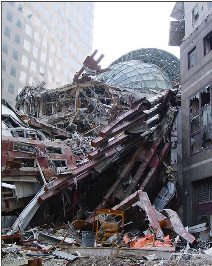
Figure 7-4 View of Winter Garden damage from West Street, with WTC 1 debris leaning against WFC 3.
