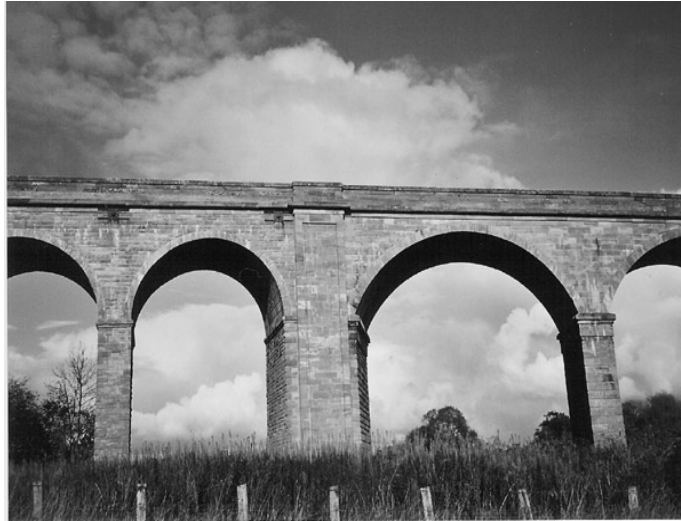
The Master Pier at the junction of the thirty-foot and fifty-foot arched spans on the Roxburgh bank © Author.
