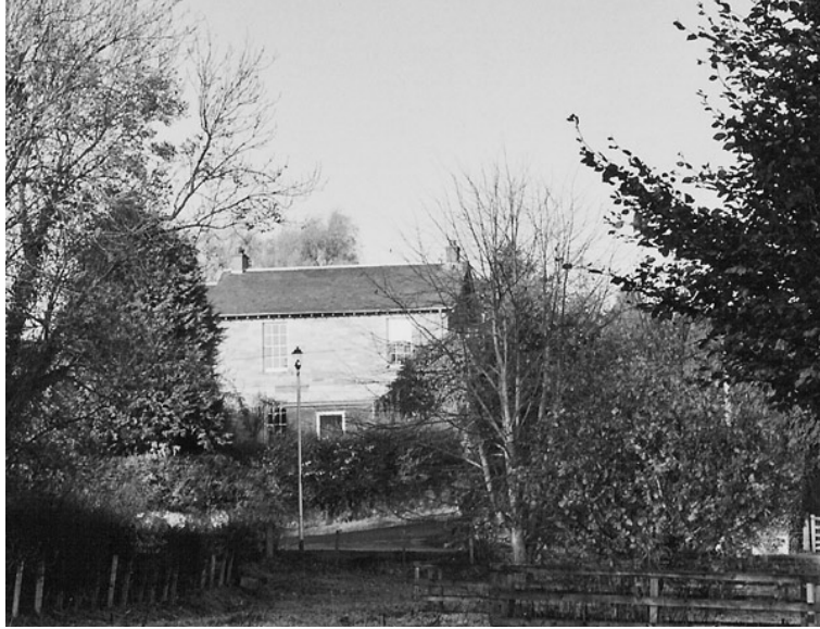
The original part of Station House 2002 © Author
