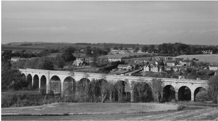
The completed viaduct viewed from Sunlaws © Author.
