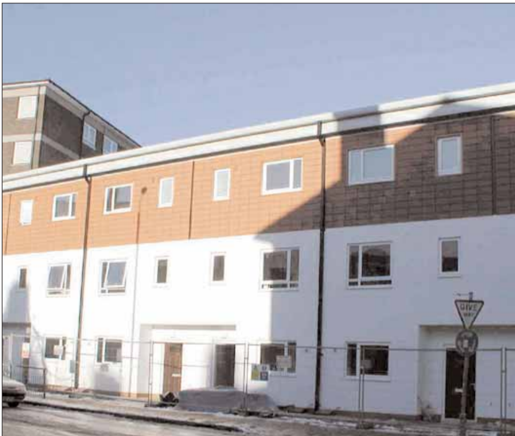
THCH put up these brand new homes in just a few weeks.
