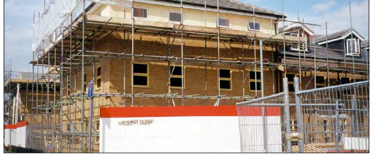
■ NEW housing association homes take shape in Stepney.
