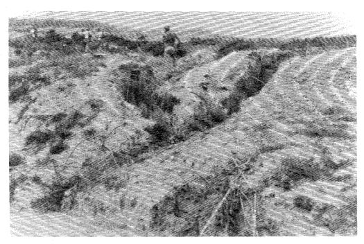
Communications trench with bamboo arches for overhead camouflage
