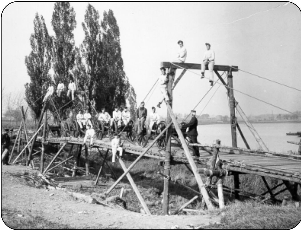
Cadets practice bridge building, 1889.
