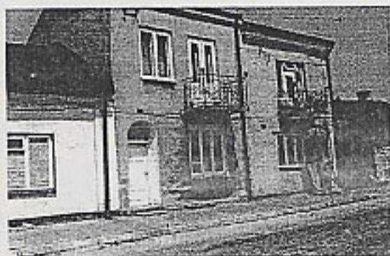
A typical street in Stopnica
