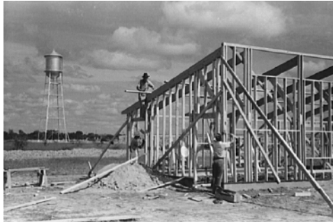
Erecting a framework.
