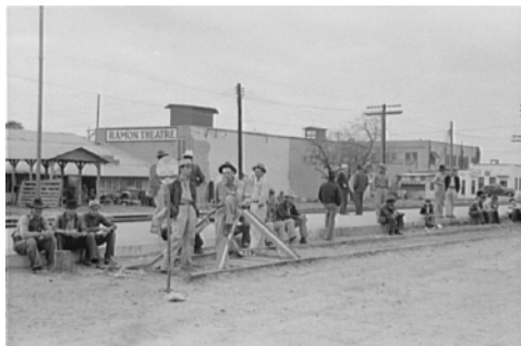
Day laborers waiting to be assigned work, Raymondville, Texas, 1939.
