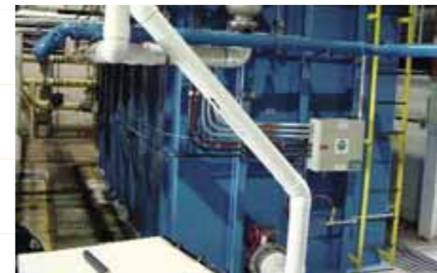
Toyota Motor Manufacturing, Kentucky, Inc., in Georgetown, Kentucky, tested a new wastewater recycling system during 2003, and found the results so positive that a permanent system was installed in early 2004. The new system significantly increases wastewater recycling at the plant, which reduces the amount of water that must be purchased from utility companies.
