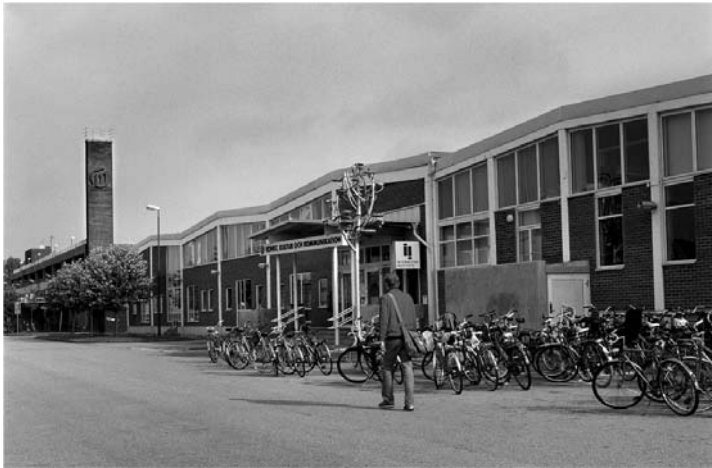
Figure 1. Exterior of the School of Arts and Communication
