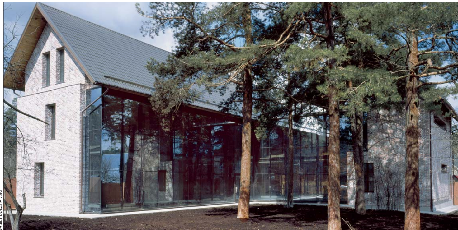
At first sight, it is difficult to make sense of just how old or how big Dmitry Geichenko's 'House with a History' is — which is exactly what the architect intended.
