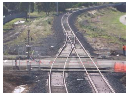
The second track, widened level crossing and new turnout
