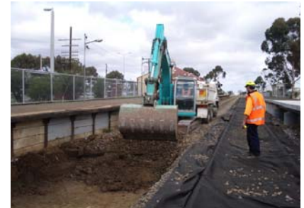
Excavation works at Melton
