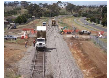
Hi-rail tipper pours top ballast at Station-Exford crossing
