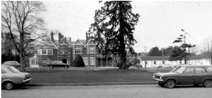
Figure 7 Bletchley Park as it is now. Two original wartime huts can be seen on the right.
