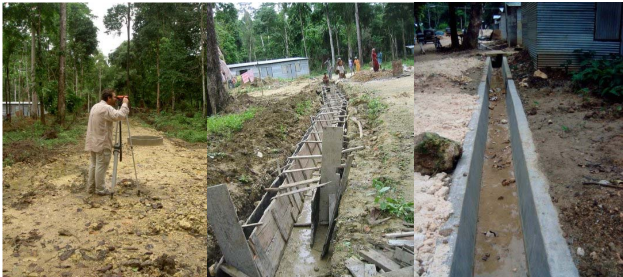
FIGURE 2 SURVEYING AND CONSTRUCTION OF SITE DRAINAGE IN HUTBAY, LITTLE ANDAMAN ISLAND
