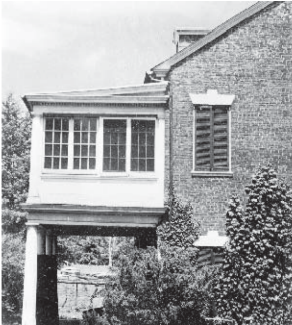
The two-story sleeping porch added by the Smoots circa 1918-1921, as depicted in a 1959 Historic American Buildings Survey photo.
