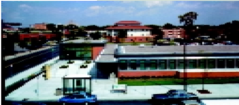
The new 5th Precinct upon completion.
