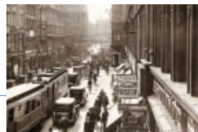
As early as the 20s and 30s Munich's streets began to fill up with traffic: Theatertinerstraße in bygone days.
