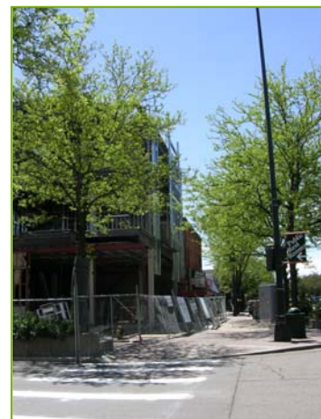
Fort Collins, Colorado (Pedestrian-friendly streetscape—top; Downtown lofts under construction—bottom).
