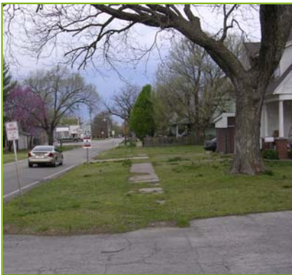
Main Street width (top); Inconsistent sidewalks and street trees, Residential Neighborhoods (bottom).
