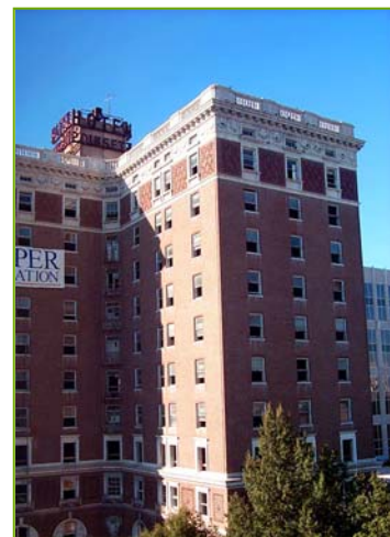
Downtown housing—Greenville, South Carolina
