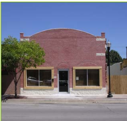
Renovation underway—Main Street
