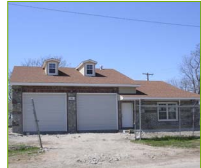
Outdoor storage and incompatible garage structure (top); Recent downtown neighborhood infill (bottom).
