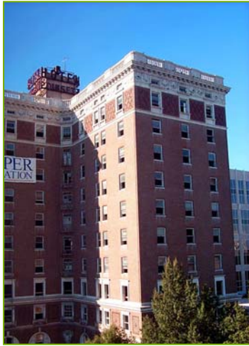
Downtown housing—Greenville, South Carolina
