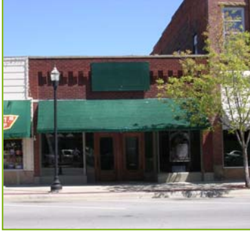
Future home of Nouveau Chocolates—undergoing renovation, 2004.
