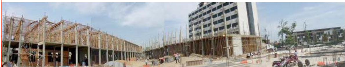
Construction of the New Building in Phnom-Penh
