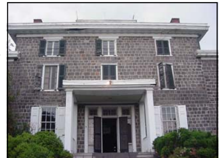
The property includes this main house and exquisite gardens designed by Marian Coffin. Preservation Delaware has been working since 1995 to protect the property. While the gardens have been restored, an appropriate reuse is being sought for the house.
