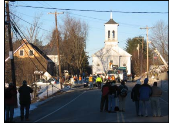
The electric wires are lowered as the Freewill Baptist Meetinghouse in Epsom, NH, makes its way down NH State Route 4 early in the morning to its new location.
