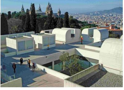
the roof and skylights and compromise the interiors. The surfaces of the poured concrete forms are failing at a rapid rate due to the rusting of the reinforcement bars, and many sections of the frameless sheets of glass have cracked or broken as the adjacent concrete decays. The Joan Miró Foundation is the youngest building on the Watch List, and it is hoped that its inclusion will help extend its life.
