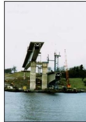
Side Span Lift
