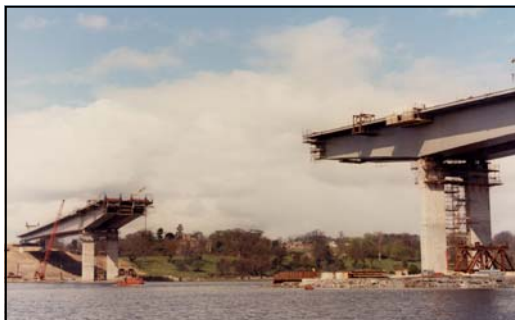
Side Spans in Position
