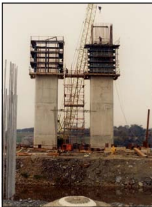
Pier Shuttering and Steelfixing Tower
