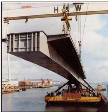
Side Span Loadout
