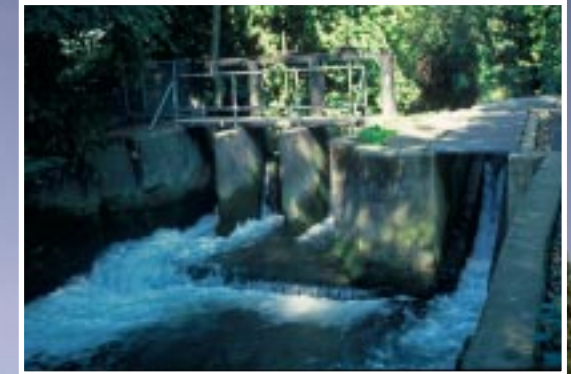
Sluice and fishpass, Bishopstoke
