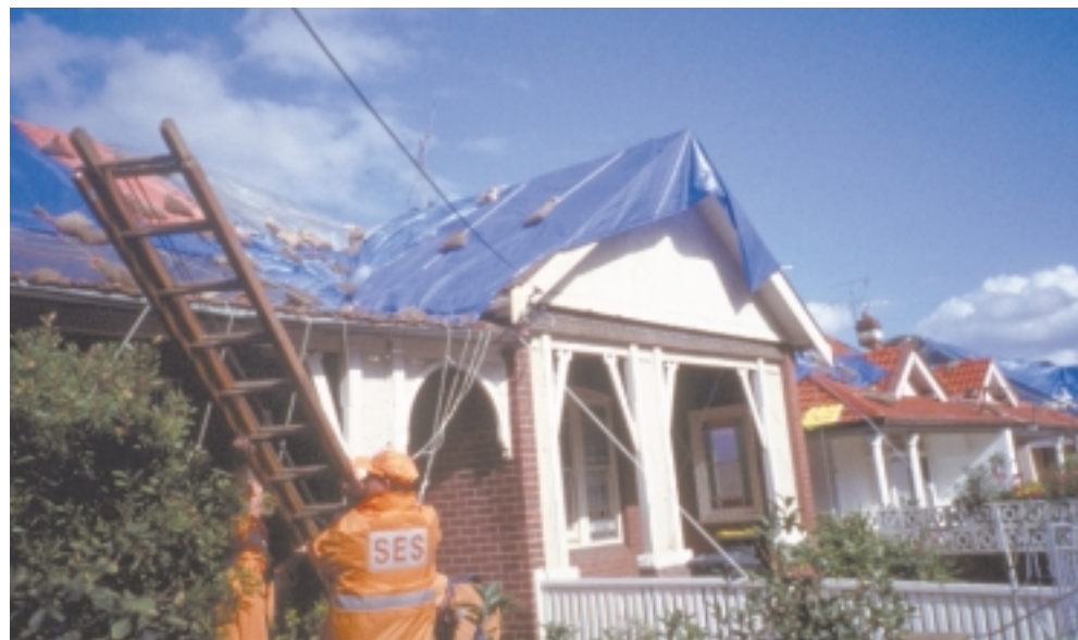
REPAIRING SEVERE STORM DAMAGE, SYDNEY, APRIL 1999.
