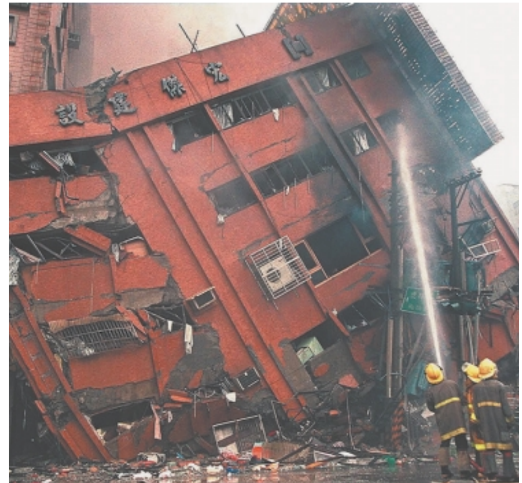
SEVERE DAMAGE CAUSED BY THE TAIWAN EARTHQUAKE, SEPTEMBER 1999.
