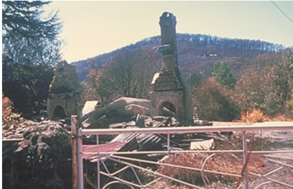
DAMAGED HOUSE. ASH WEDNESDAY BUSHFIRES, 1983.
