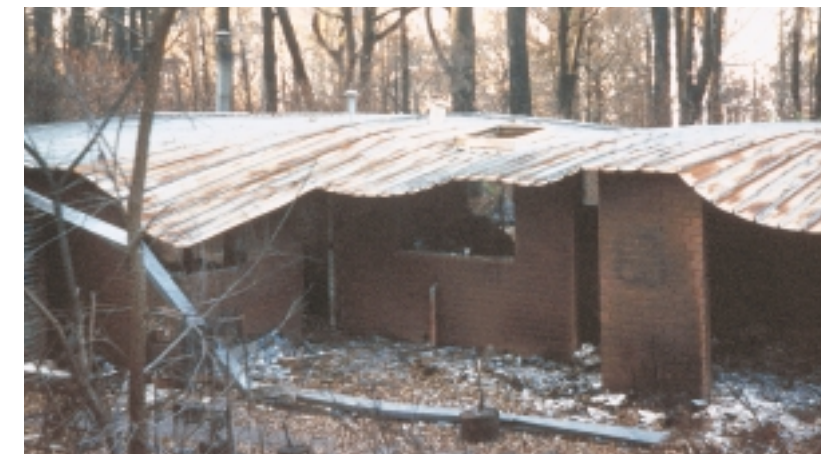
HOME DESTROYED IN DANDENONG BUSHFIRES, VIC. 1997.
