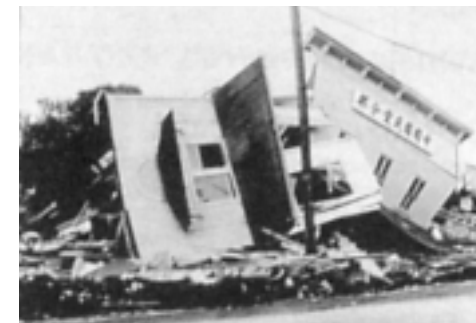
TSUNAMI DAMAGE, OKUSHIRI ISLAND, JAPAN, 1993.
