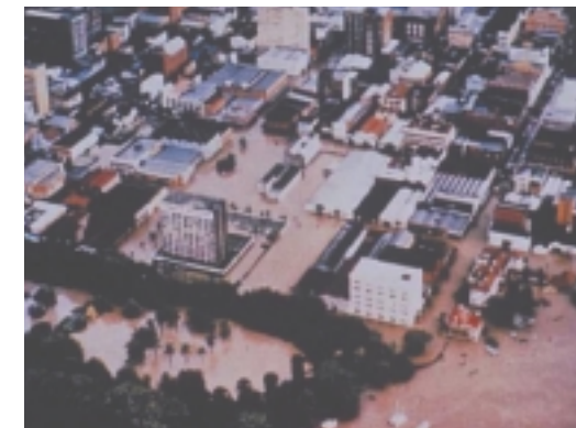
INUNDATED CBD, BRISBANE RIVER FLOOD, 1974.
