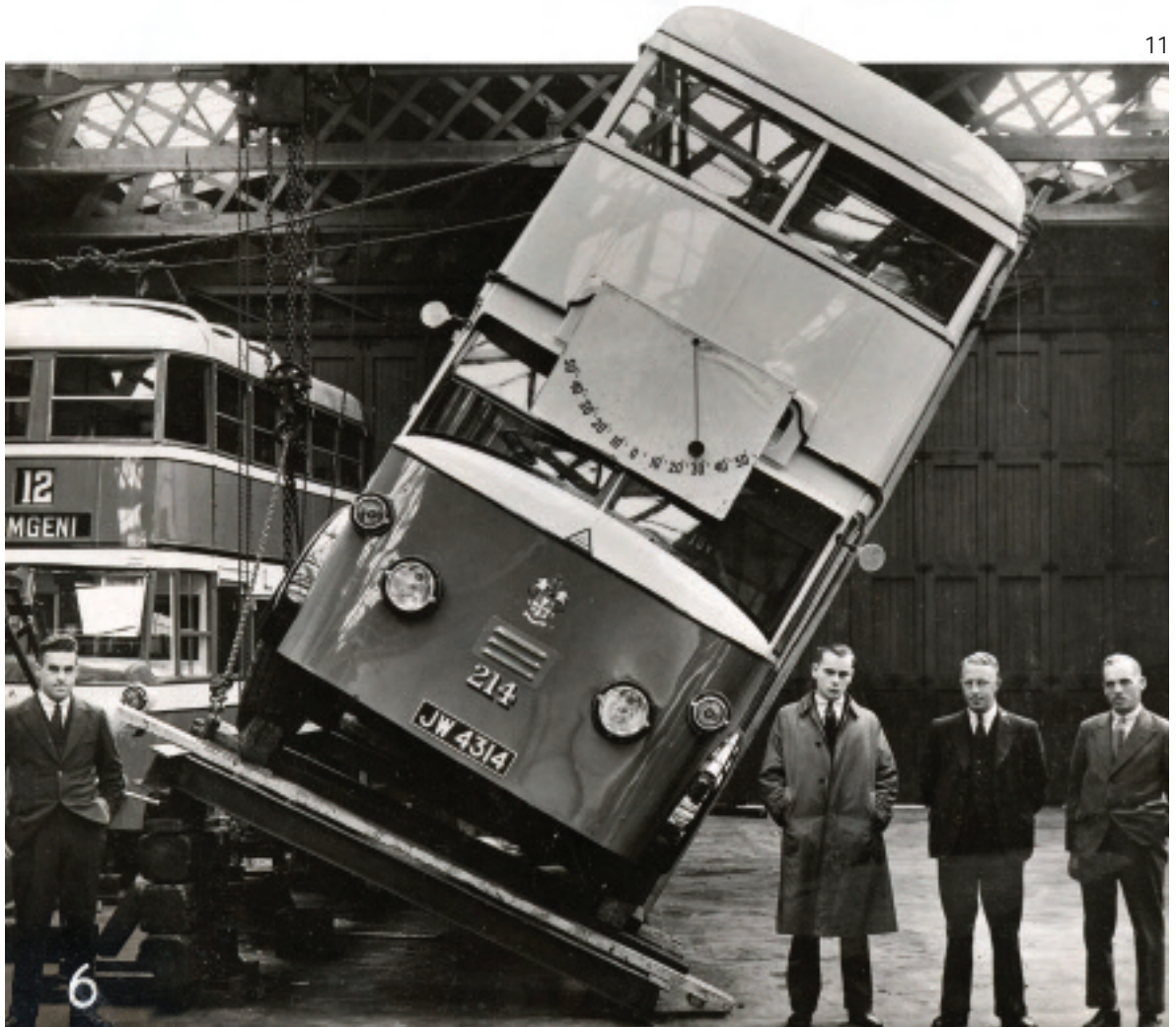
11 A tilt test of a new Sunbeam trolley bus, built in Wolverhampton in 1934. (Wolverhampton Archives and Local Studies, P/3549)
