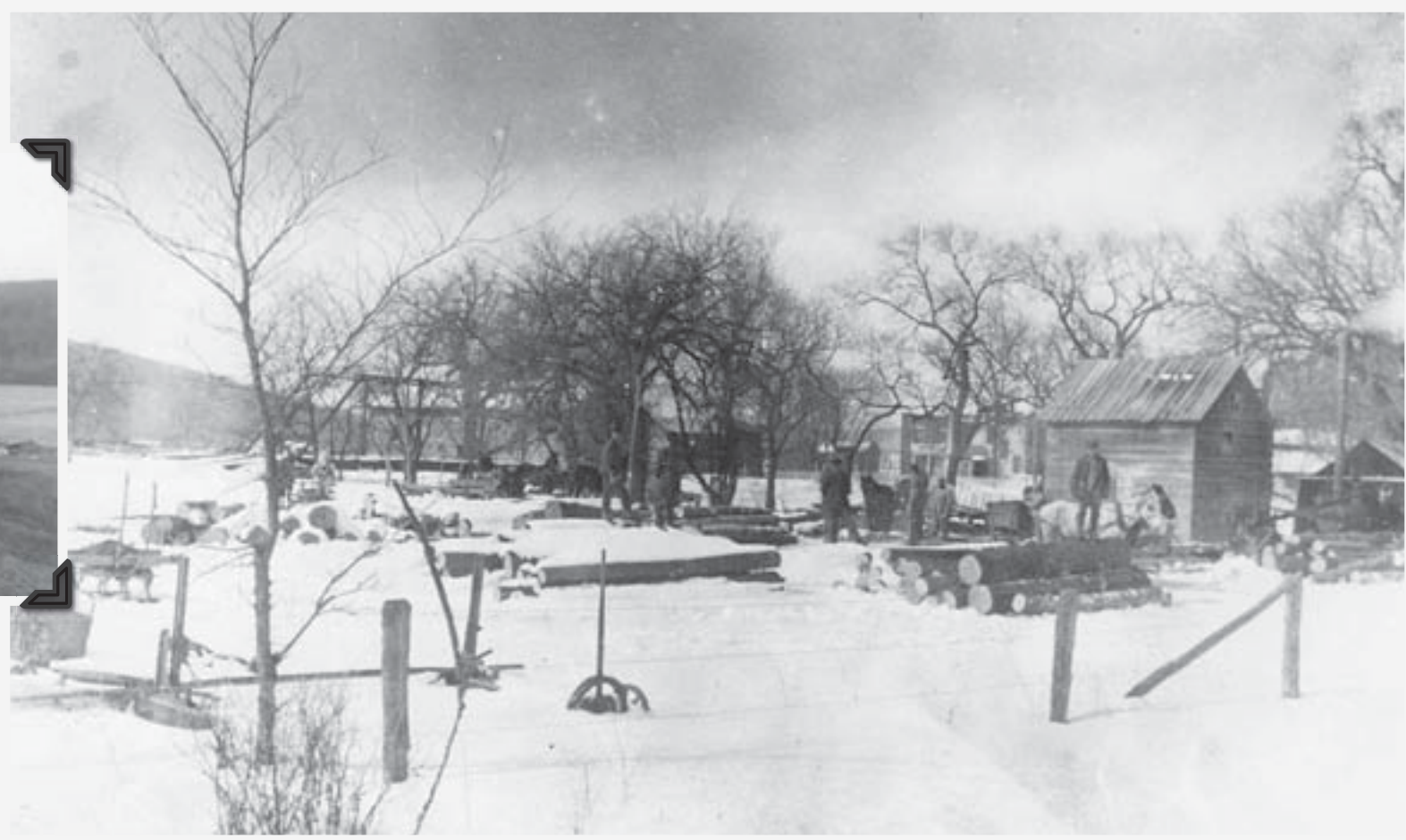
The Meighen and Luedtke sawmill. Powered by a steam engine, the mill helped meet the huge demand for lumber in Forestville's early days.
