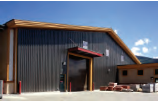
DOE/NREL, PIX 09173, Jim Yost
