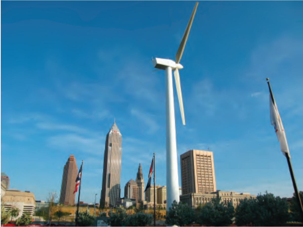
The wind turbine on the front lawn of the Great Lakes Science Center in Cleveland, Ohio, helps increase public awareness about renewable energy, and provides an estimated 7 percent of the building's annual energy needs.
