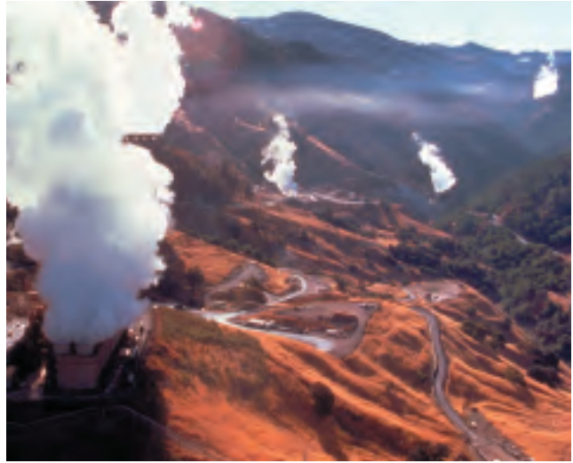
DOE/NREL, PIX 00060, Pacific Gas & Electric
