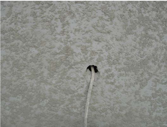
Figure 14: Electrical utility installed after water management system
