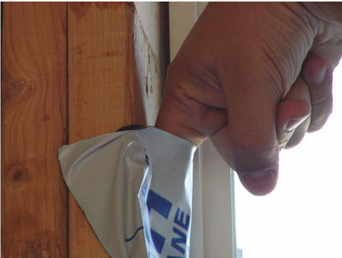
Figure 29: "Fishmouthing" of the membrane
