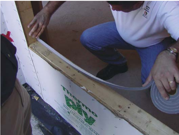
Figure 31: Weather seal gasket used as a backdam
