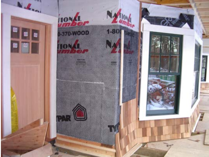
Figure 5: Drainage matt installed behind wood shingles
