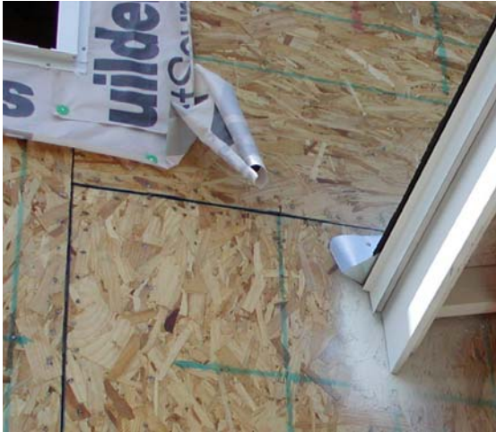
Figure 12: Kick out flashing installations
