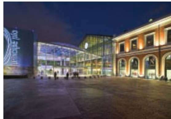
Renovation or Expansion of an Existing Project 1 Yorkdale Shopping Centre Toronto, Ontario (Canada)
