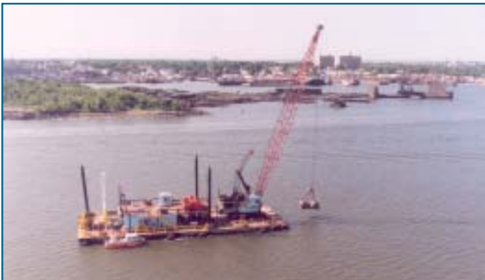
A massive fleet of dredges, drill boats, scows, and other work boats is currently working on three major channel deepening and several berth deepening projects in the New York/New Jersey harbor. (Photo above) The 41-foot deepening of the Arthur Kill Channel, where it joins with the Kill Van Kull and Newark Bay just north of Howland Hook began this summer. Work is also under way south of the Goethals Bridge in a portion of the channel that serves tankers and other bulk ships. (Above right) Work is continuing towards a 2004 completion date for the 45-foot deepening of the Newark Bay Channel, just off the wharf of the Elizabeth-PA Marine Terminal. (Right) Work began earlier this year on the deepening of the Port Jersey Channel to 41 feet. Port Jersey serves the Auto Marine Terminal (foreground, right) and the Global Container Terminal (background, right). On the left is the former Military Ocean Terminal in Bayonne, NJ, now known as The Peninsula at Bayonne.
