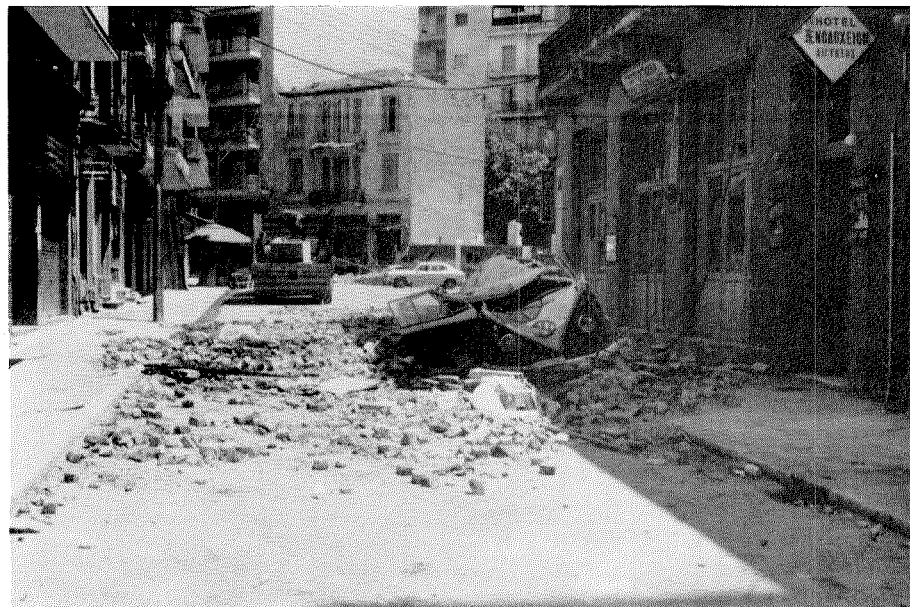
Figure 11. Damage to the parapet walls and the balconies of "Egyptos" Hotel.
