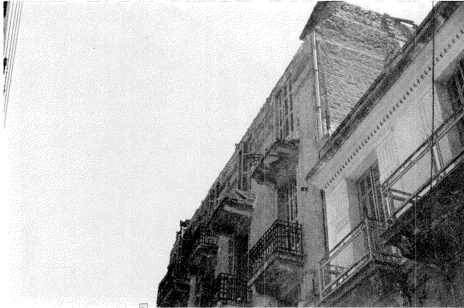
Figure 11. Damage to the parapet walls and the balconies of "Egyptos" Hotel.
