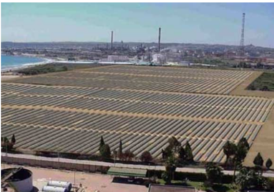
FIGURE 11.11 Archimede plant as envisioned at the site of ENEL power plant in Priolo Gargallo (Sicily, Italy).
