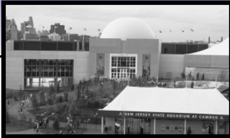
NREL/PIX/07329 NEW JERSEY STATE AQUARIUM
