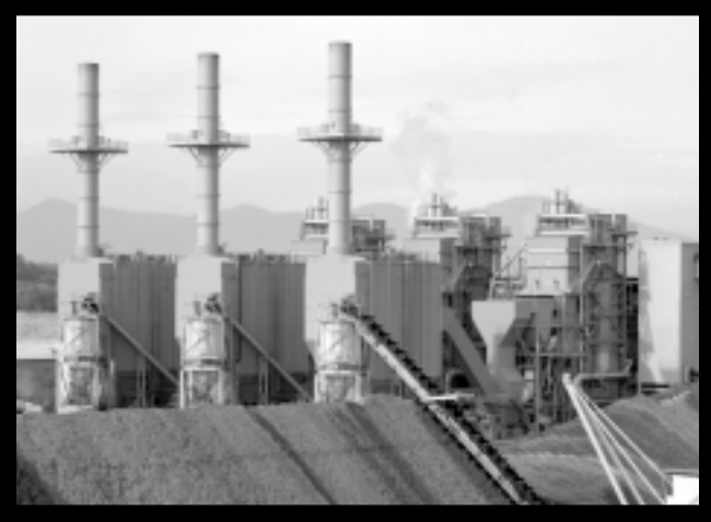
This 50-MW biomass power plant located in Anderson, California, runs on residues produced by nearby companies in the forest products industry.
