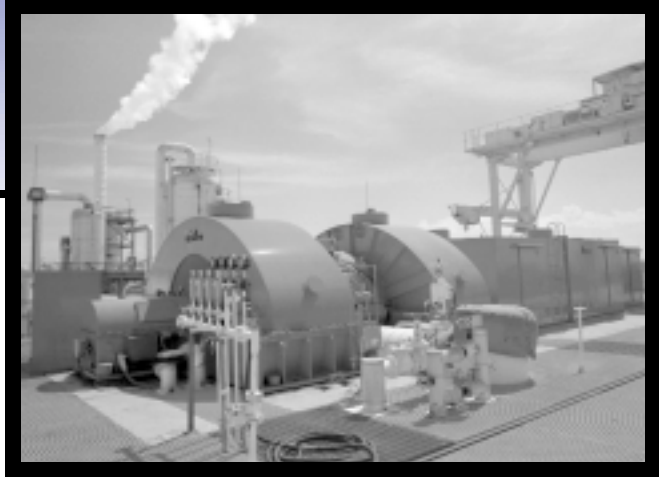
This geothermal power plant located in the Imperial Valley in Southeastern California generates electricity from steam produced underground in the Salton Sea Geothermal Reservoir.
