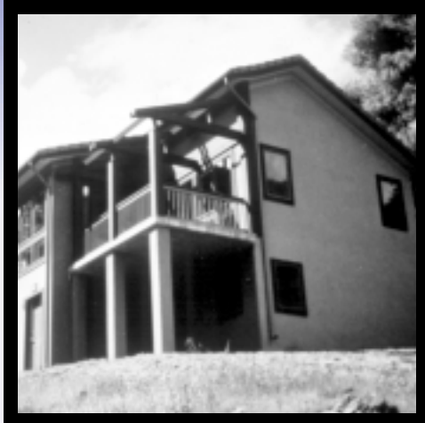
This home for Park Service employees at the Grand Canyon in Arizona incorporates solar design with a Trombe wall, structural insulating panels, high-performance ENERGY STAR® windows, an integrated mechanical system, and ENERGY STAR® appliances, reducing the annual heating need by more than 90%.
