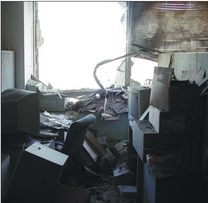
Figure 6-12 Office at the north side of the 8th floor.
