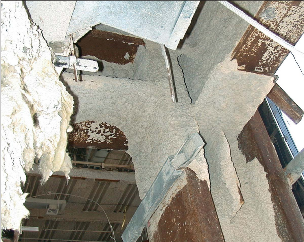
Figure 6-6 Moment-connected beams to columns.
