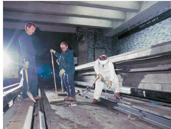
Track maintenance carried out at night by métro trackmen. (STM Archives)
