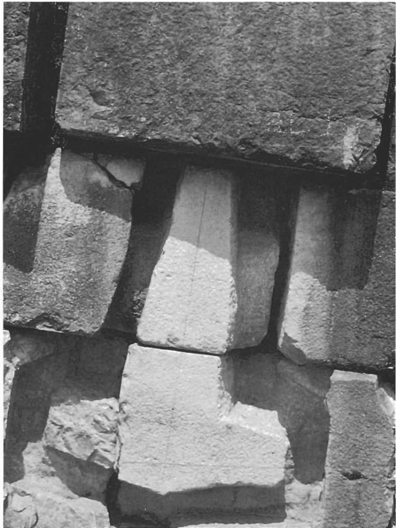
70 One of the sockets in Augustus' naval monument at Nicopolis. It held a ram somewhat bigger than the Athlit ram (Figs 59–60), perhaps from a 'six'. Late 1st century BC.
