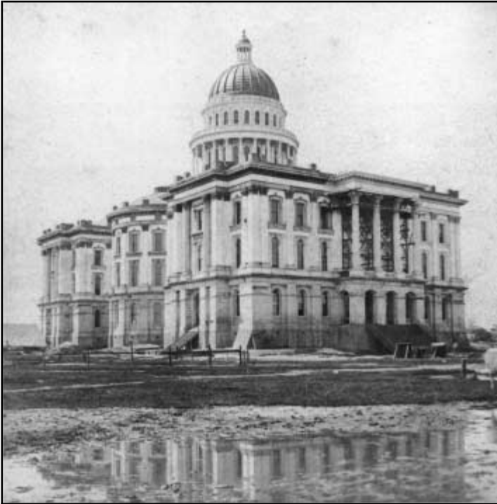
Capitol nearing completion, circa 1872
