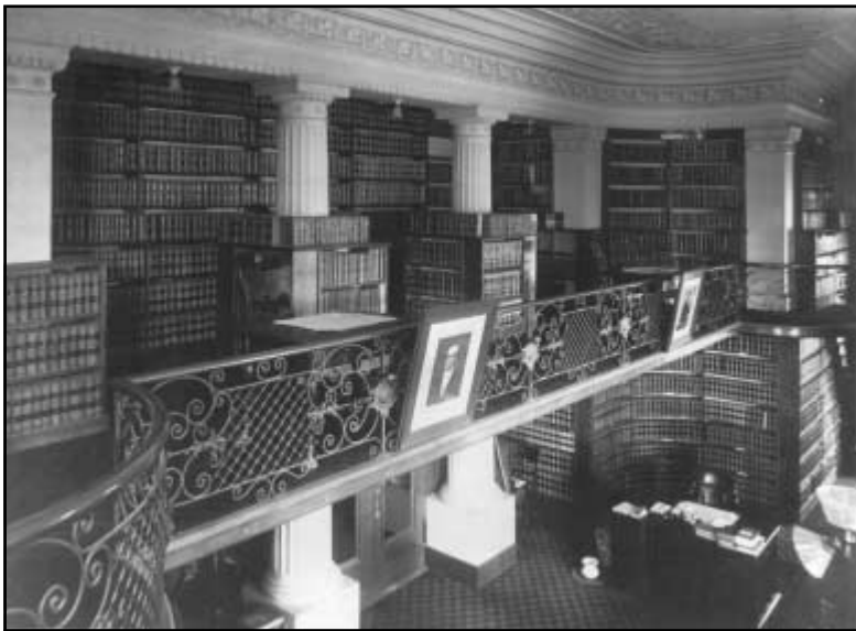
State Library, Law Department, 1904 (replaced Supreme Court Chambers in apse)
