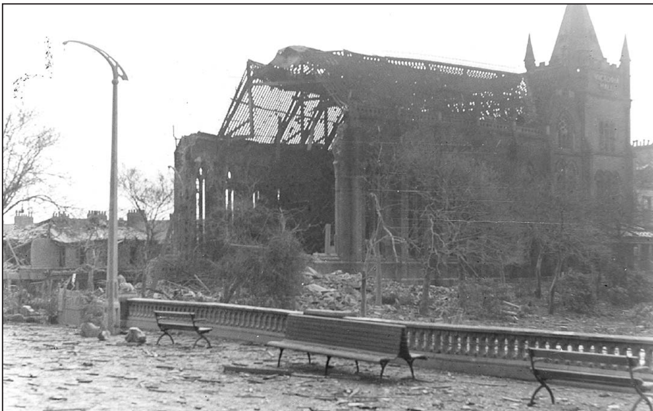
The bomb damaged Victoria Hall in 1941
