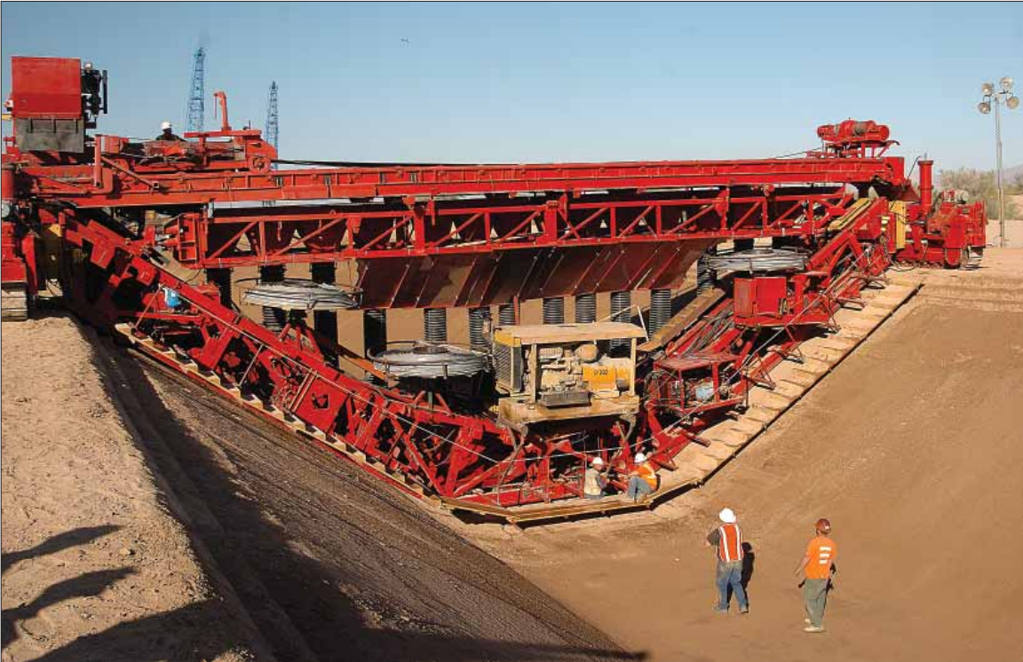
Right: Workers calibrate the paving machine to ensure it meets its specified tolerances. The paving machine pours the concrete lining onto the dirt canal.
