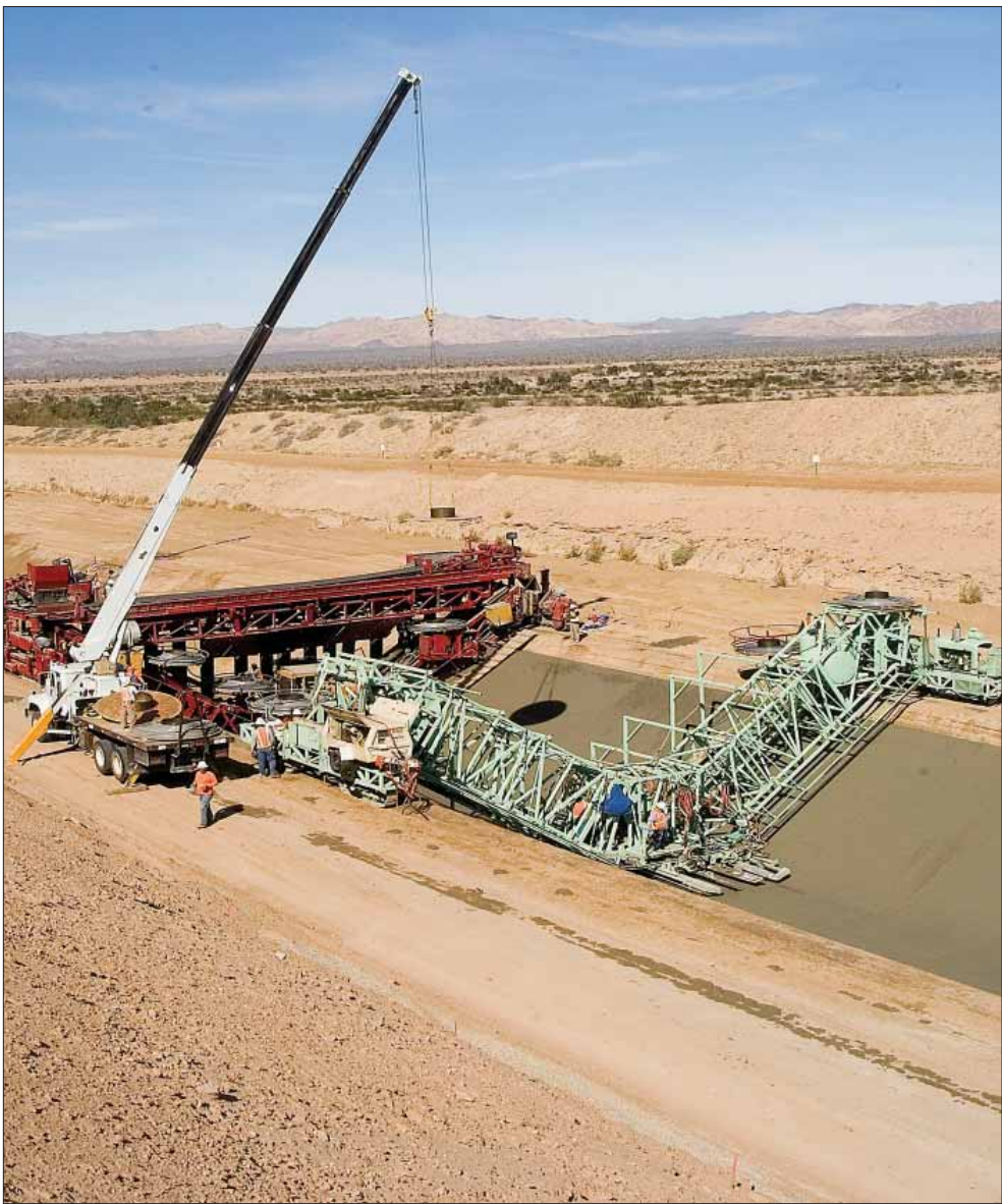
Right: Workers calibrate the paving machine to ensure it meets its specified tolerances. The paving machine pours the concrete lining onto the dirt canal.
