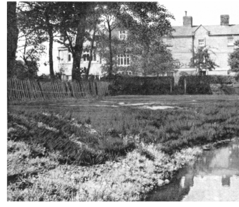
Bromborough Court House
