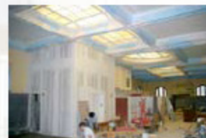
Original skylights restored at Franklin
