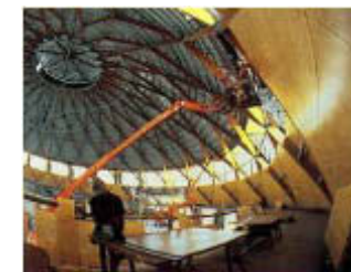
23. The wood and metal framing in the Dome's interior has ignited widespread architectural interest 24. Shafts inside the cattle pavilions allowed effective mechanical ventilation
