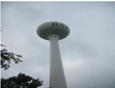
Figure 4: Phase 2 WiMAX antenna location
