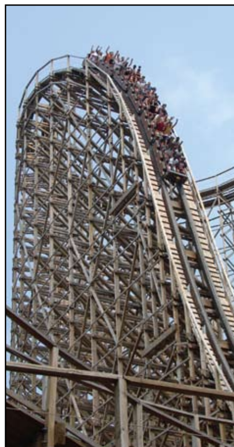
AT PHOTO/TIM BALDWIN
