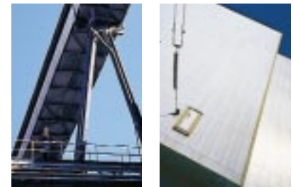
Tarong Power Station's coal supply conveyor belt (left) and turbine hall.
