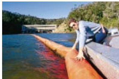
Peter McGuigan routinely inspects the oil booms at Wivenhoe Power Station.
