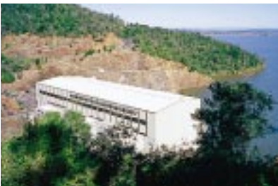
Wivenhoe Power Station is Queensland's only pumped storage hydro power plant.
