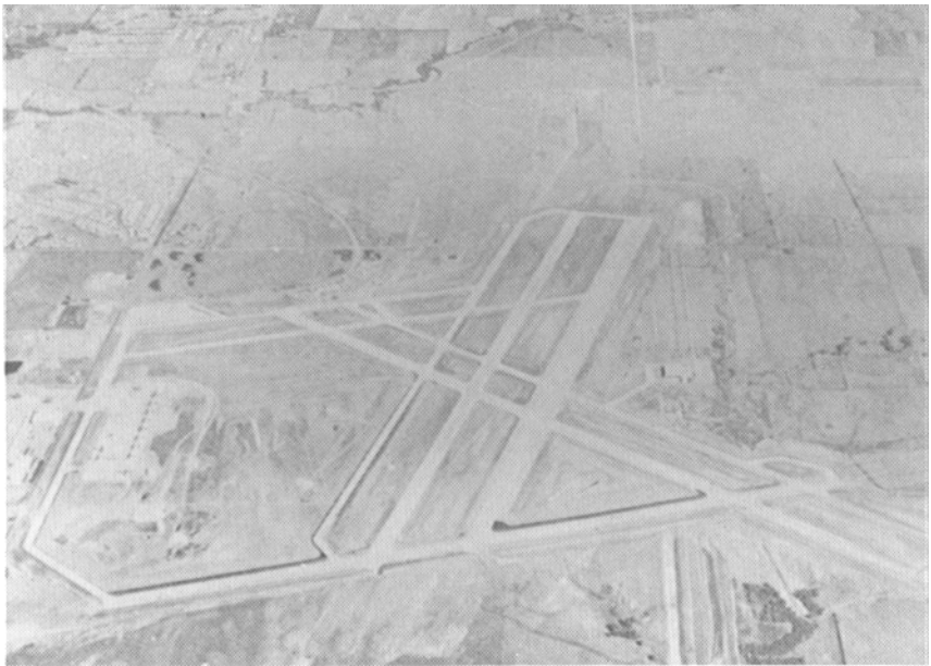
Wichita Municipal Airport, October 1943
